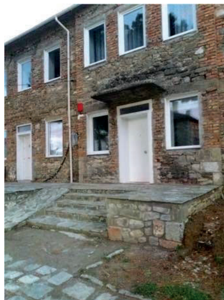
Figure 3. Ramps in Health Center in Erseka
