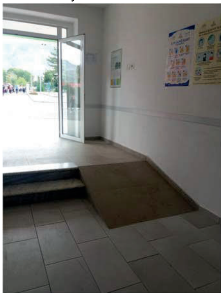
Figure 2.Ramps photo in Secondary School in Erseka.
